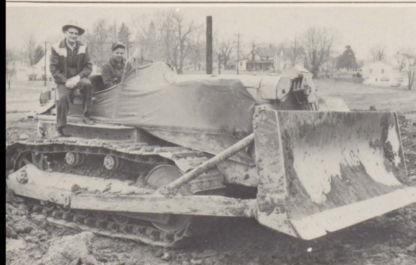
Claude Sullivan and his helper perch atop a bulldozer. C.C. SULLIVAN EXCAVATOR AND CONTRACTOR Phone Wilson 8-4797
