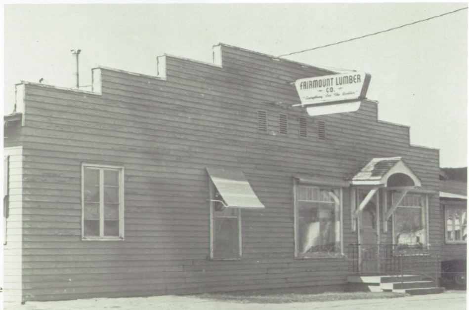
Fairmount Lumber has "Everything for the Builder."
